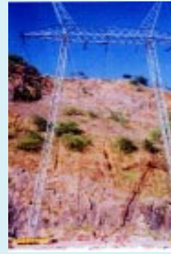
Analytical and Experimental Investigations on 400 kV Portal Type Guyed Towers
