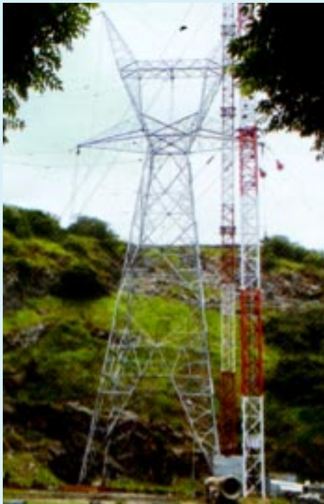
400 kV S/C Tower Type “TL-30” - M/s Gam Arak Company, Iran
