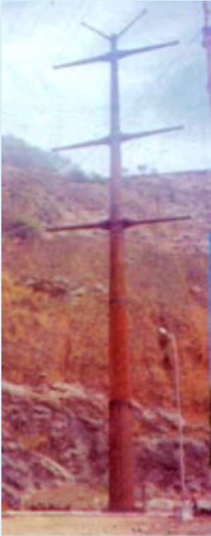
400 kV D/C pole at test bed
